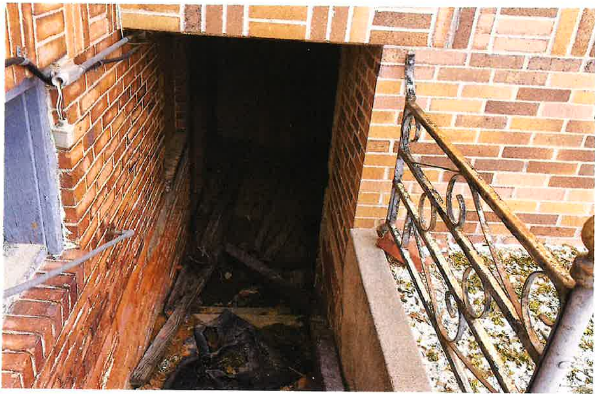
1107 Central Ave. December 28, 2018 Exhibit 1, pg. 3
