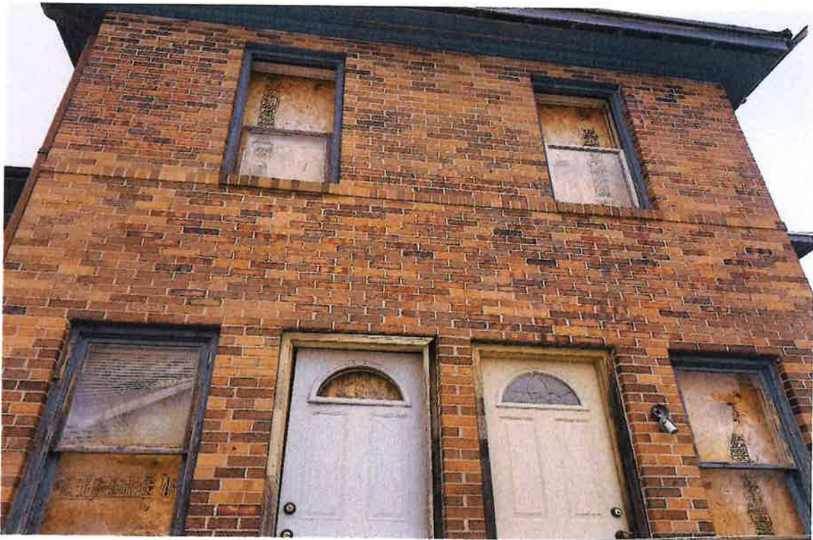
1107 Central Ave. December 28, 2018 Exhibit 1, pg. 1
